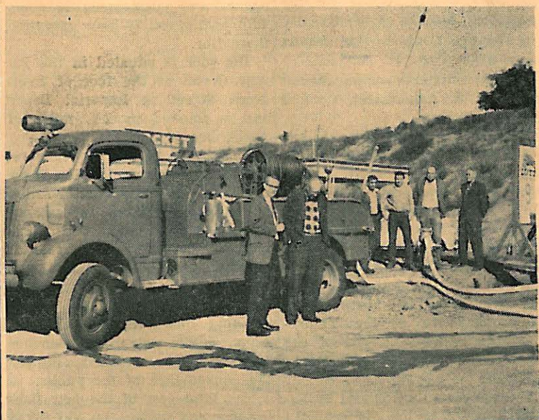
Alpine Volunteer Fire Department personnel test new fire hydrant installed recently east of the Rocket Service station on Highway 80. Volunteer fire hydrant truck shown testing water service from fire hydrant. From left, Ed Houser, Engineer-Manager of Rio San Diego MWD; Orville Palmer, Fire Commissioner; George Brant, volunteer fireman; Mace Bratt, volunteer fireman; Jack Blankenship, Chief of the Volunteer Fire Department, standing directly behind fire hydrant; and Phil Hall, Fire Commissioner and volunteer fireman. Echo Photo
